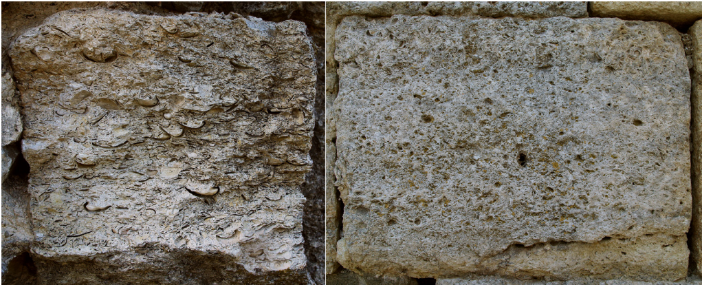
Fig. 10. Blocks of sandy limestone in the pediment of the temple of Jupiter (left) and in the wall of the west entrance zone (right), macroscopic appearance (photo: B. Djurić)
