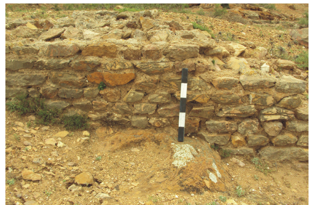
Fig. 11b. Green schist and antique yellow rubble stones used to build construction walls (photo: A. Younès)
