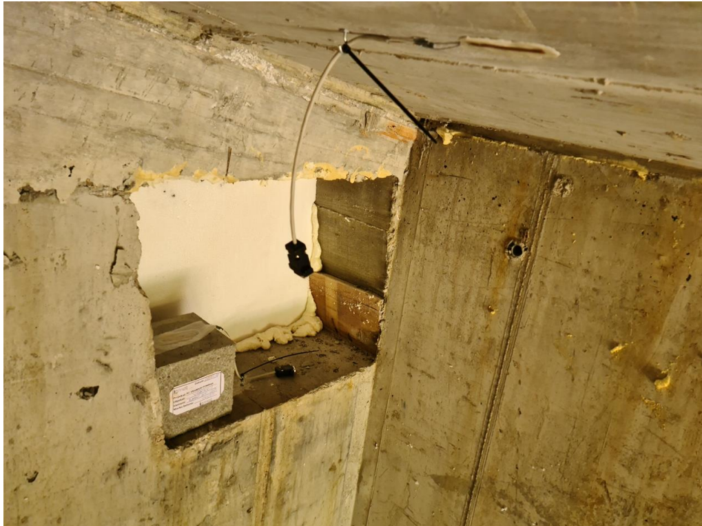
Figure 46. Strain gauge on a concrete sample used for temperature compensation
