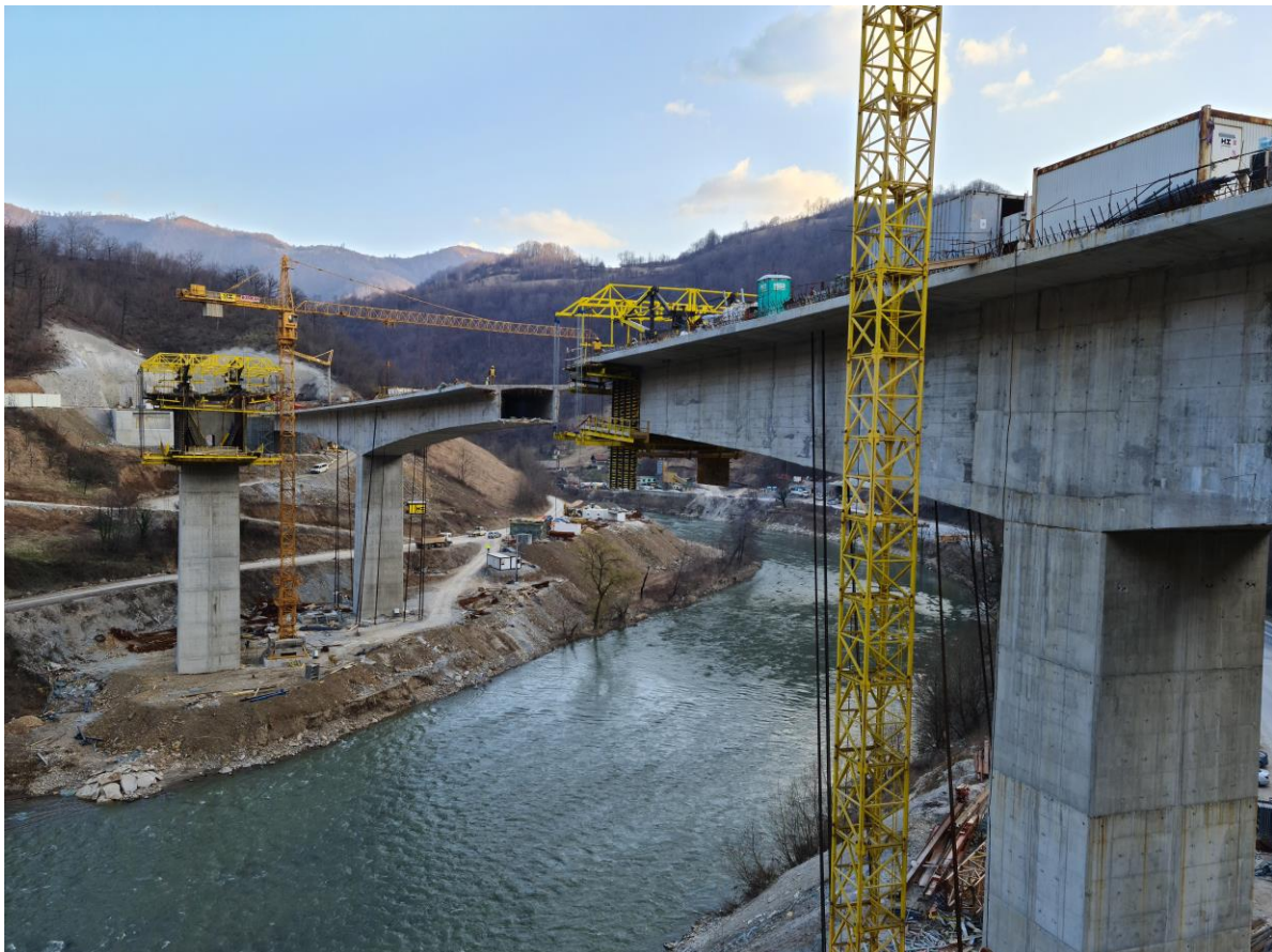
Figure 37. Vranduk 2 bridge under construction
