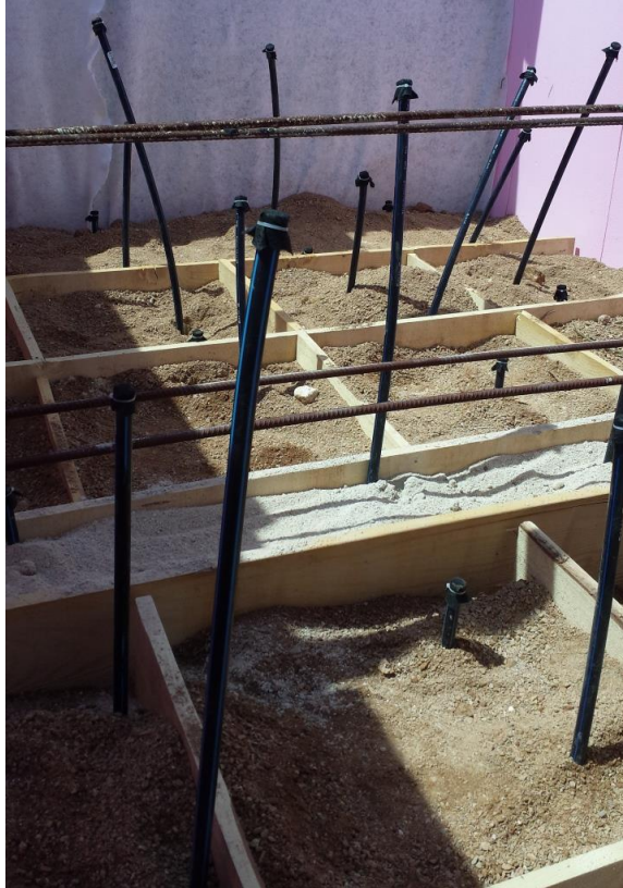
FIGURE A.5: Filling the material.
