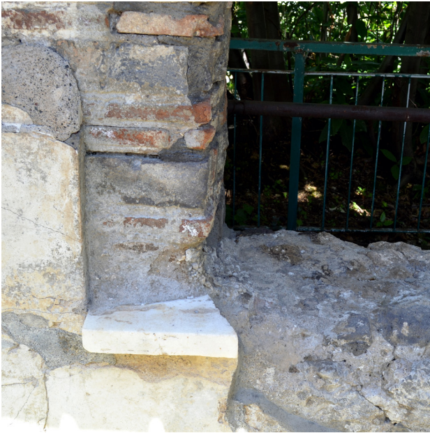
Fig. 10. Stabiae, Villa Arianna, Room P, garden window sill with non-Italian white marble (photo: J. Clayton Fant)
