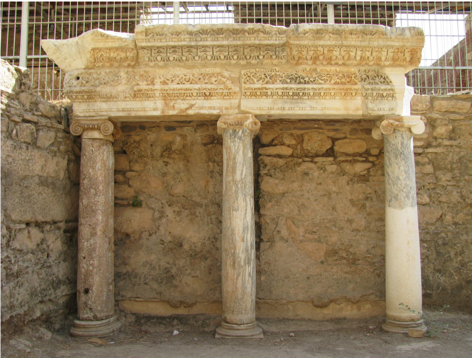
Fig. 4. The restored columnatio of the proskenion
