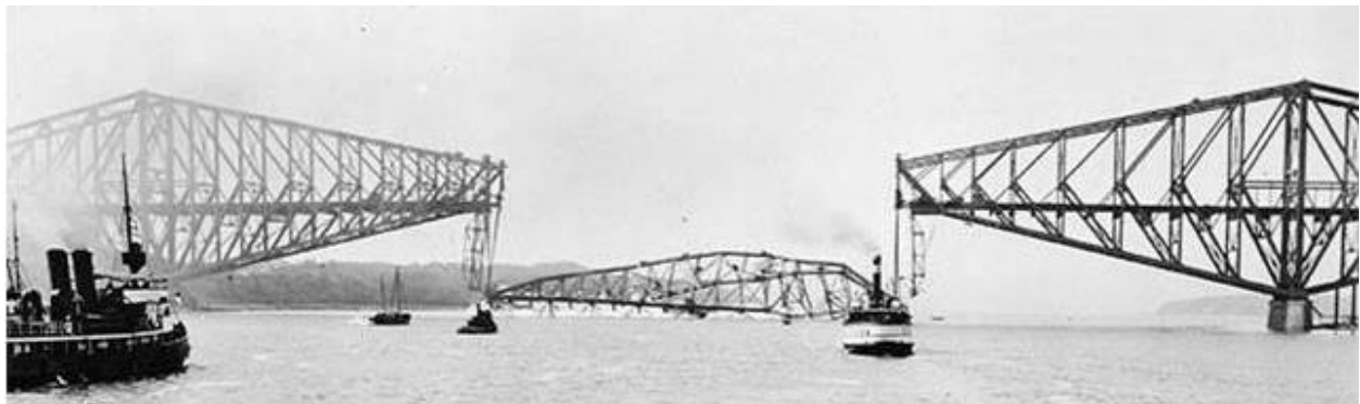
Figure 19. Quebec bridge, collapse of the central segment
