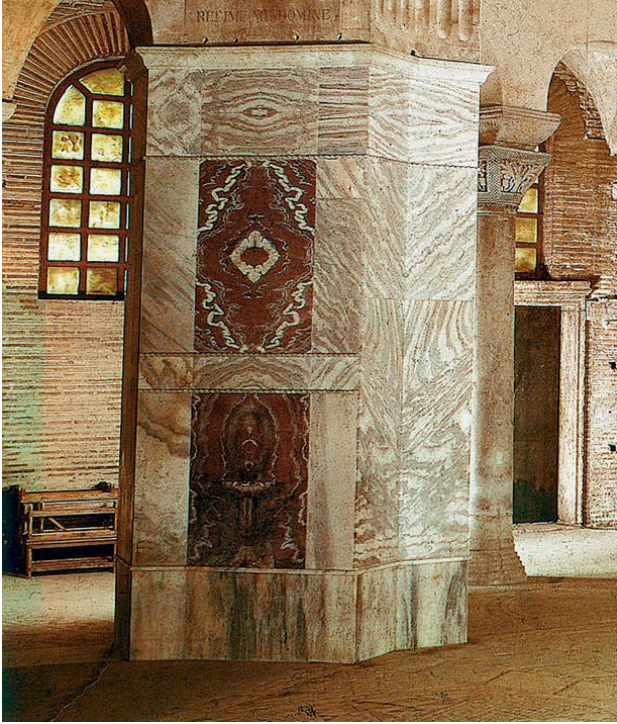
Fig. 7. San Vitale in Ravenna, wall cladding made of Iasian cipollino (photo: D. Peirano)
