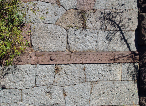
Fig. 8. Coursed polygonal masonry and horizontal decorative band at Tower I on the acropolis (photo: © Archive of Larisa)
