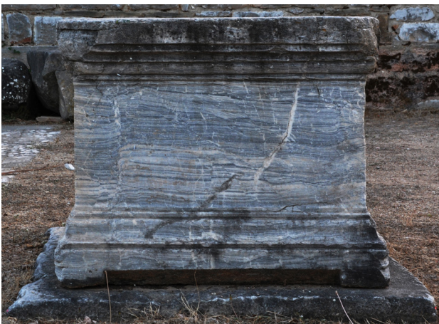
Fig. 11. Iasos, south stoa, plinth of grey veined stepped Euromos marble, n. 2, of the central piers
