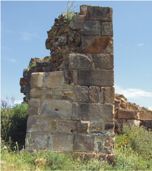
Fig. 12. Green schist squared blocks used to build a Byzantine tower (photo: A. Younès)
