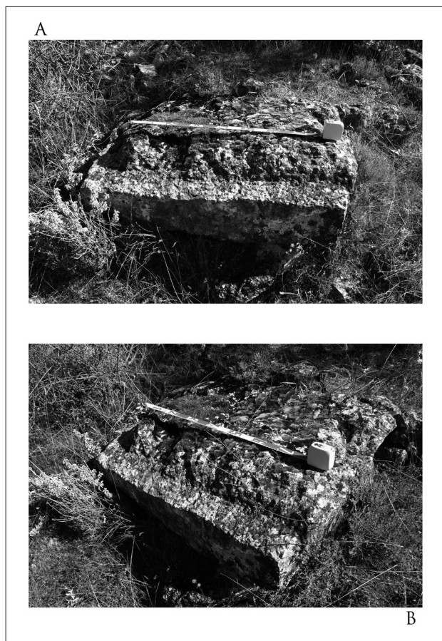
Fig. 6. Various views of one of the blocks located in the immediate vicinity of extractive area that presents different surface finishes: on the one hand, two of the perimeter edges appear finely worked with the chisel, while the central area has only been slightly roughly shaped with a pointed tool, such as a pick or a pointer
