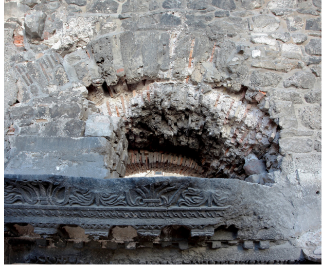
Fig. 4. Peristyle, relieving arch above the portal leading into the Vestibule before restoration (photo: Ž. Bačić)
